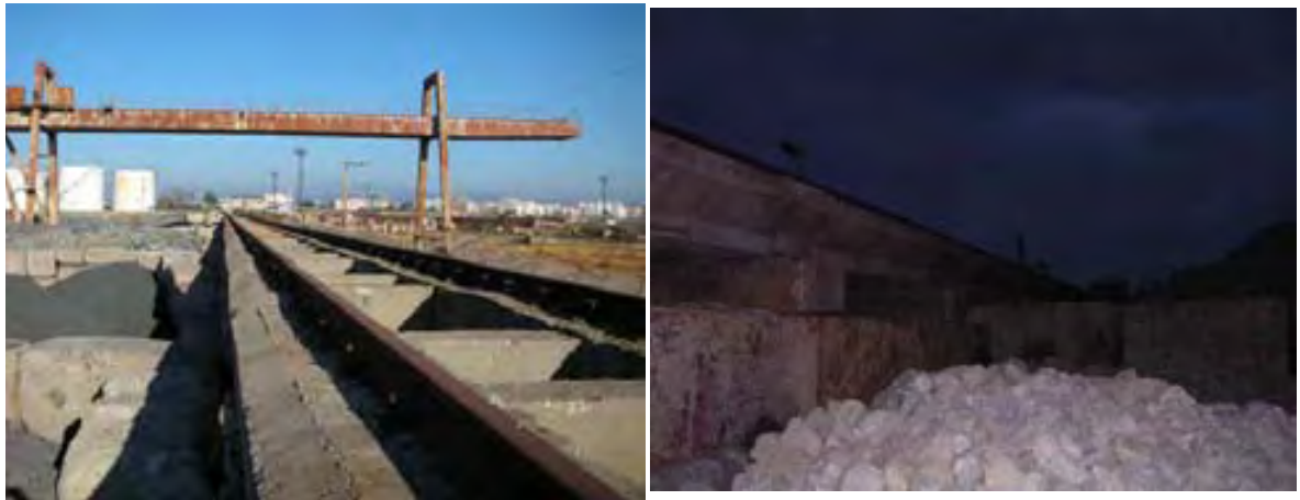
Figure 6-3 Railcar dump station with elevated track behind berth 10
