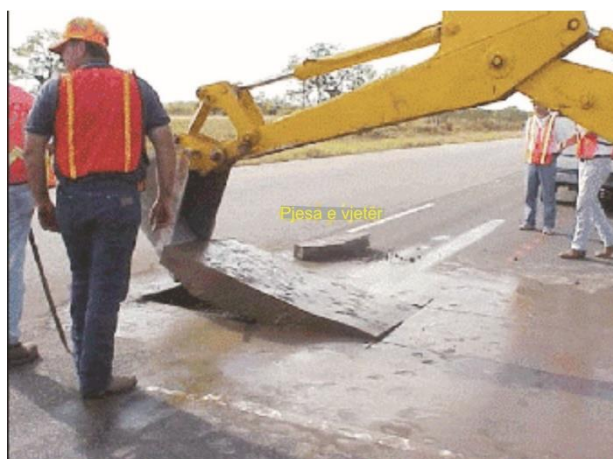
Figura 1.19: Heqja e Bllokut (Asfalto-Beton ) me prapaeskavator
